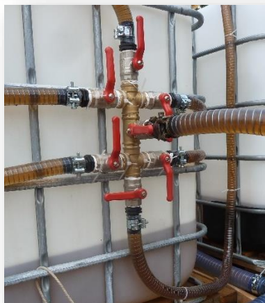
Filling GROUNDDECO into the tanks by pump and counter
