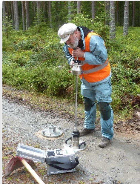
measuring of "EV dyn" [ MPa ], using 10 kg "Light Falling Weight Deflectometer"
