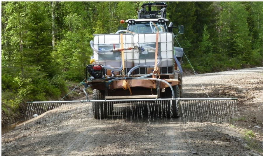
spraying a mix consisting of GROUNDECO + water on to surface
