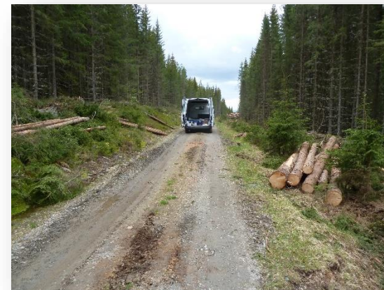
stat. 3+150 ( look back to the start of construction )
