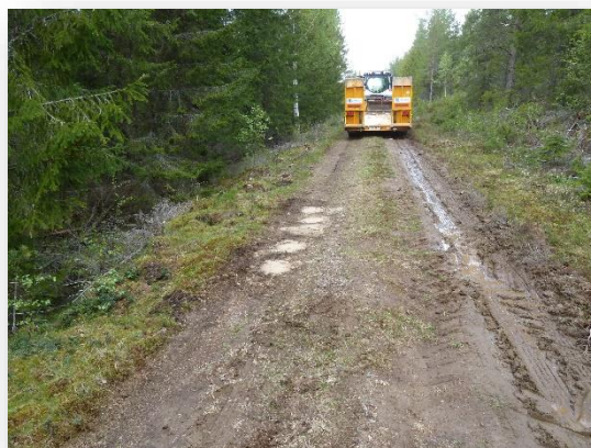
stat. 4+350 (look back to the start of construction)
