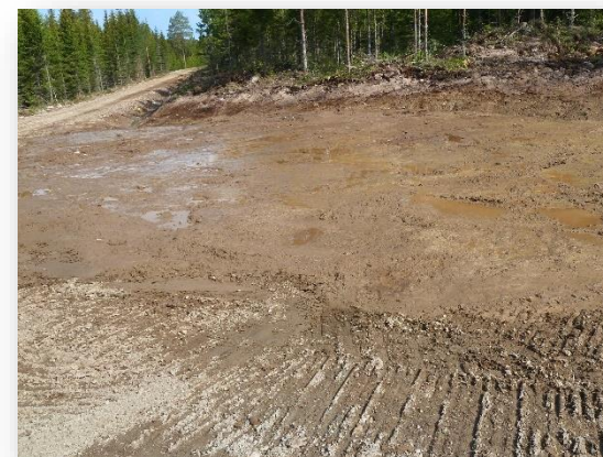
stat. 4+500 (look back to the start of construction)
