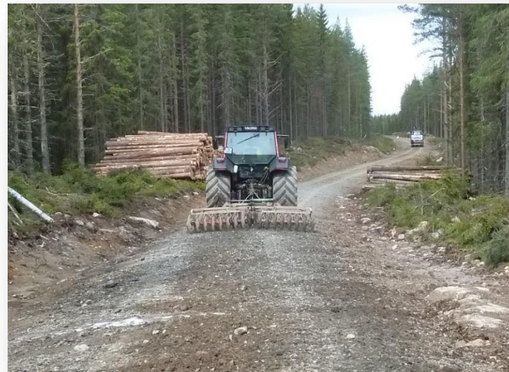
mixing and drying the soil using a disc harrow
